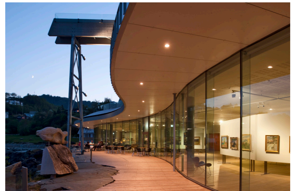
Deep recessed small downlights integrated in colonnades and canopies
