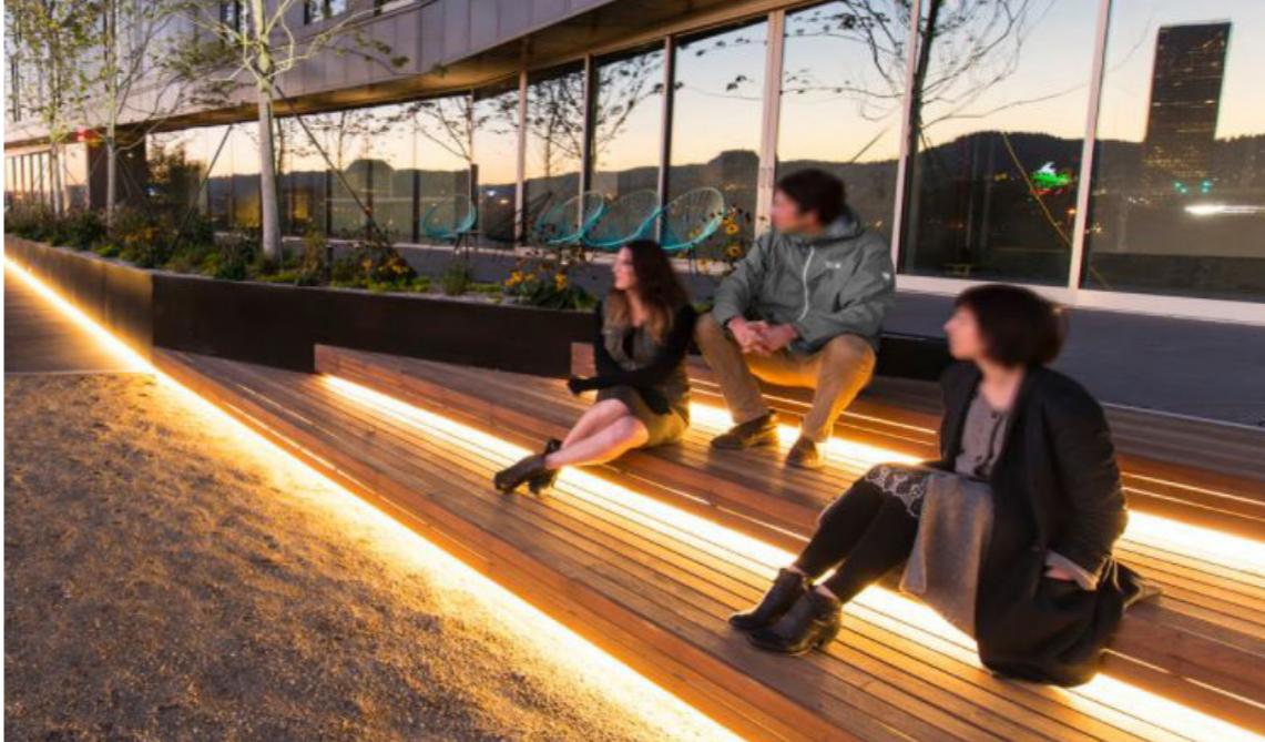
Low placed linear lights are integrated in the wooden sitting deck
