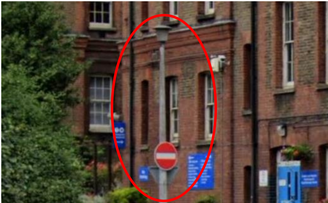
Figure 4-5 Existing Site Entrance Column Lighting
