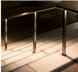
3 - LED lighting integrated in handrails.
