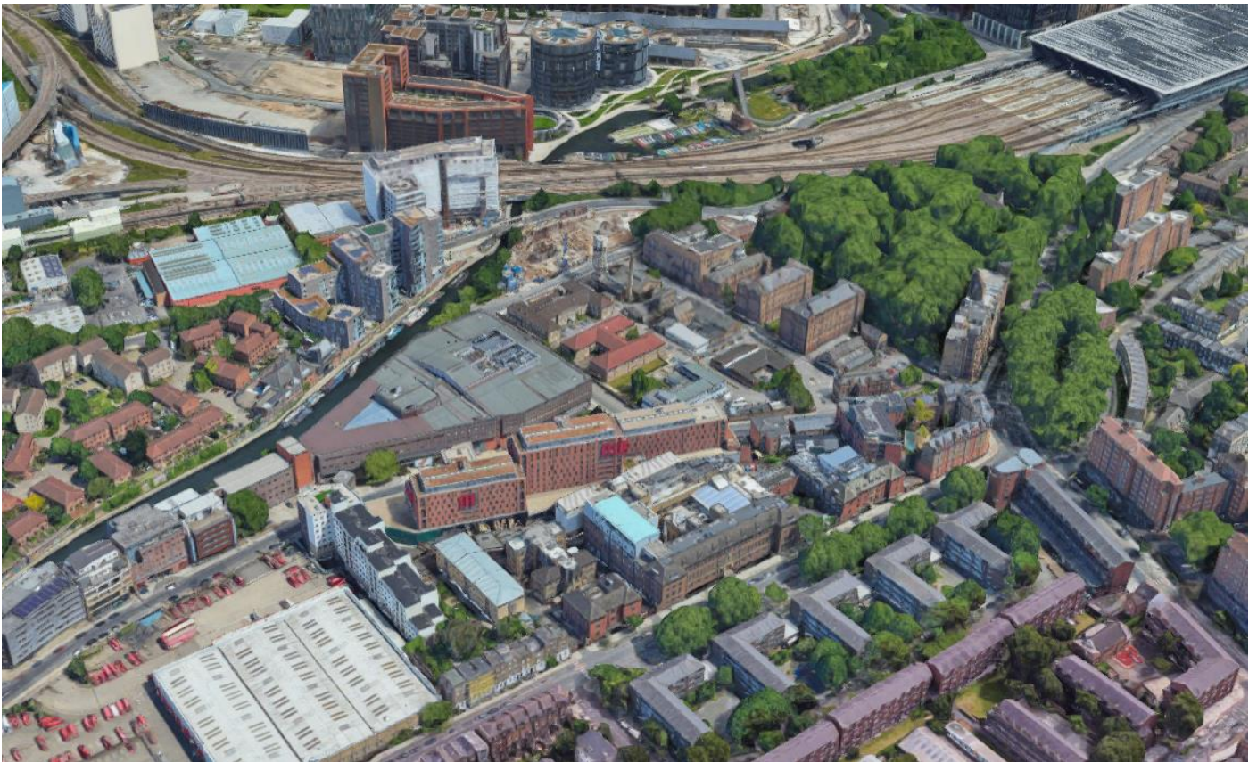
Figure 3.1: Aerial Image of the Site and Context (Source: Google)
