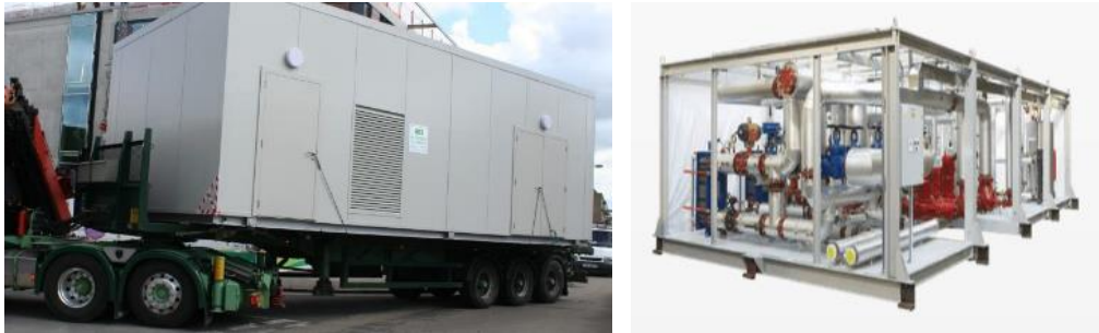
Figure 3-4 Prefabricated plant rooms
