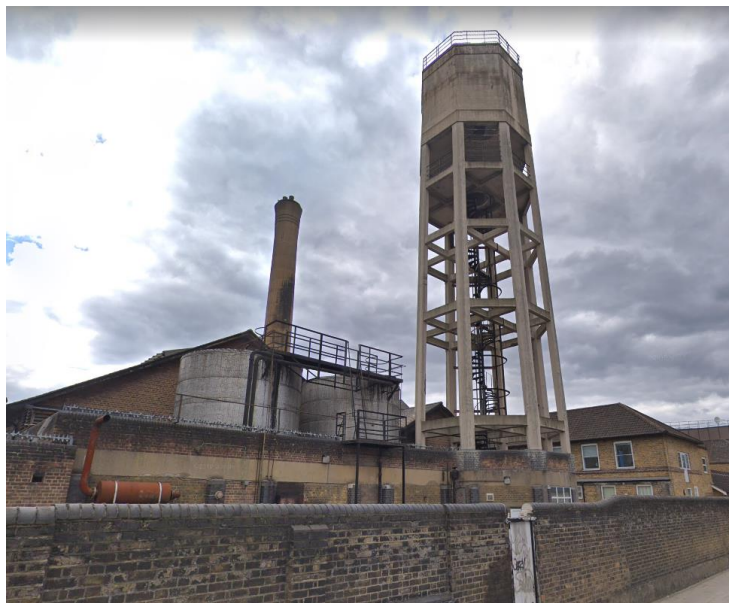
Figure 2-2 Existing Boiler House on St Pancras Hospital Site
