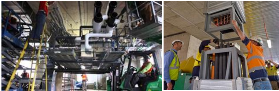
Figure 3-7: Examples of Off-Site Manufacture
