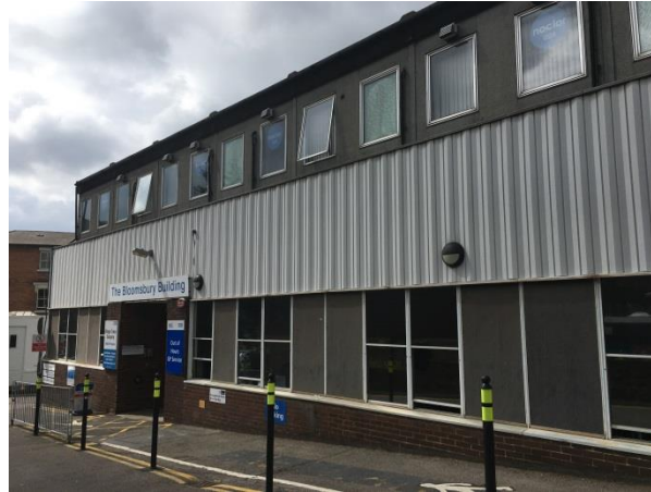
Photo 11. Southern elevation of the Bloomsbury Building (B4).
