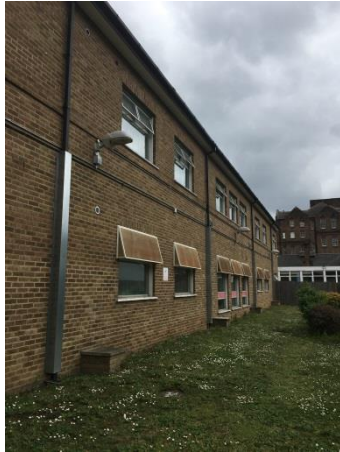
Photo 10. Eastern elevation of Ash House (B3).
