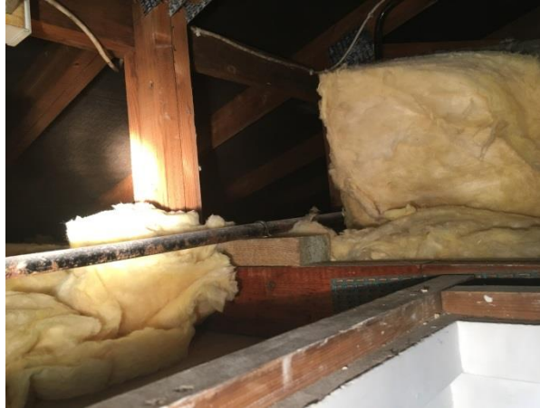
Photo 5. Roof void of Jules Thorn (B1).
