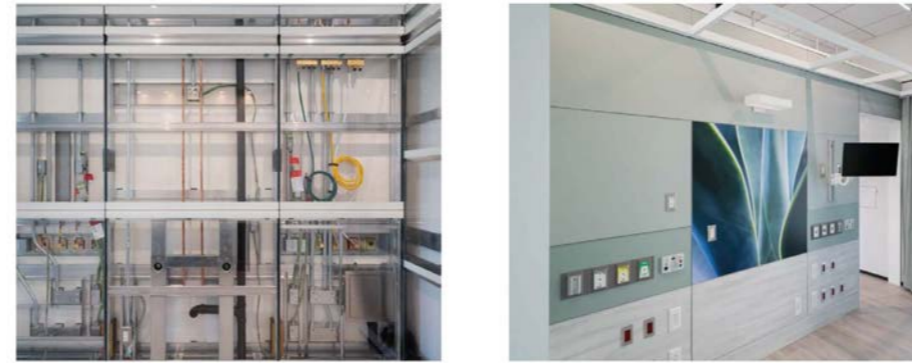
Modular systems - MEPH, partitions, structure
