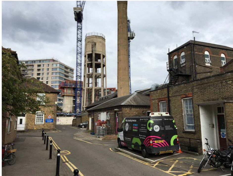
4 The kitchen building complex (on the right)
