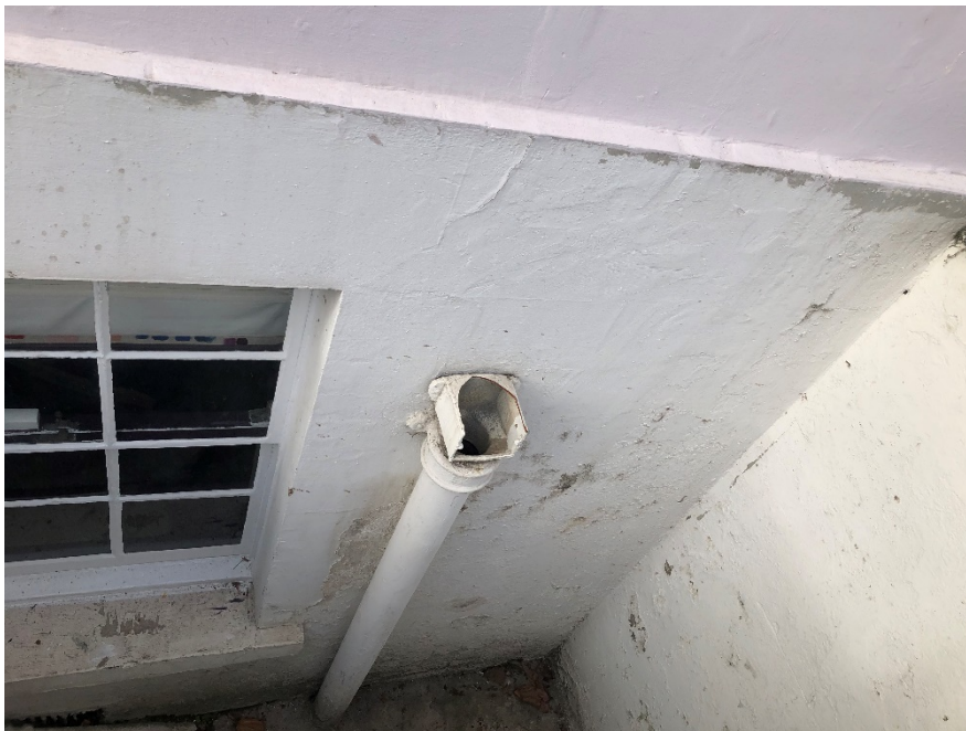
Figure 5: Broken Ventilation Pipe
