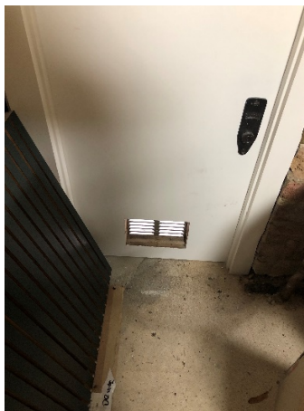
Figure 2: Existing ventilation grate in lightwell door
