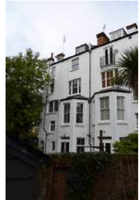
▲ Fig 5. Rear elevations of numbers 57-59 with out of character dormer windows at attic level
