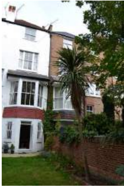
▲ Fig 6. Rear elevations of number 55 and 53. Number 53 shows original un-rendered brick elevation
