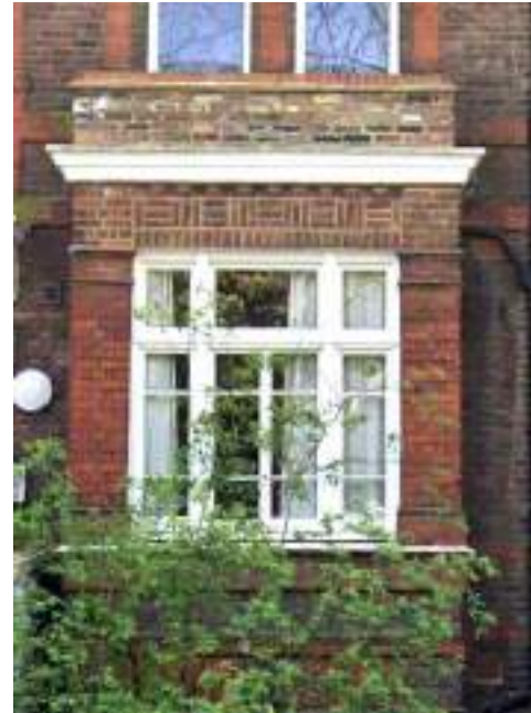
▲ Fig 4. Decorative brickwork above projecting bay window to the front of number 55
