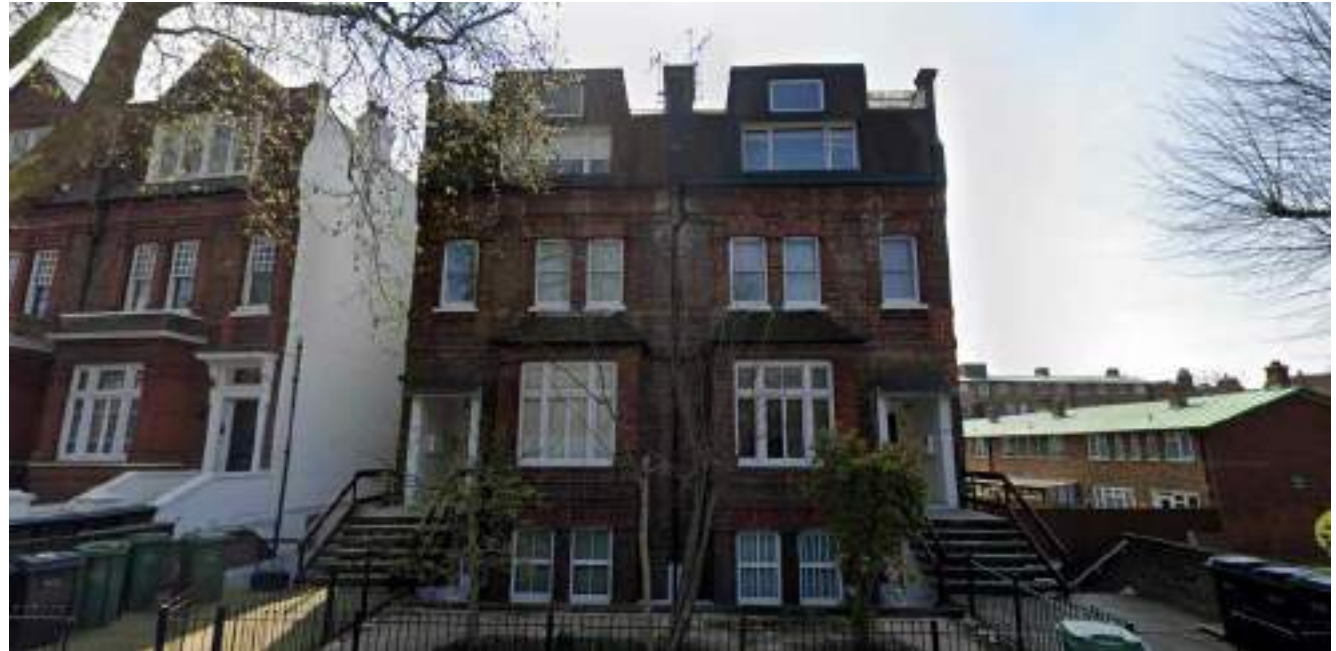
▲ Fig 7. Neighbouring property (numbers 57-59) with unsightly and out of character attic conversions. Dwellings of a different typology in the background likely date to the late 20th Century.
