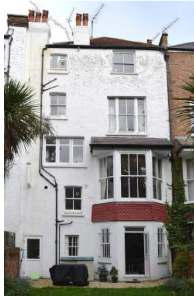
B Existing Rear Elevation Photograph
