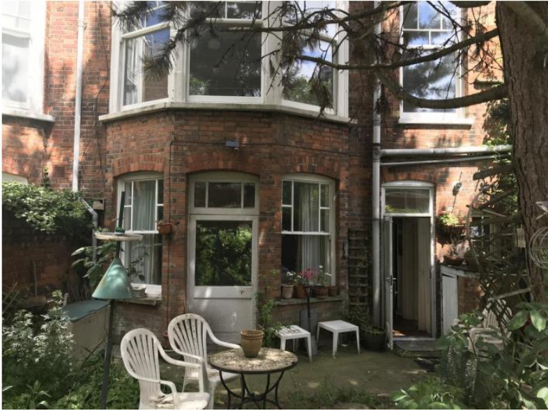
3. View of rear elevation
