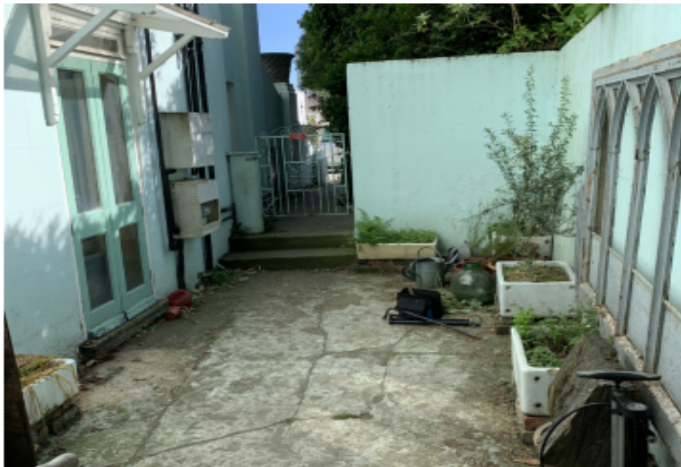
Image 2. Showing the existing neighbouring boundary wall.
