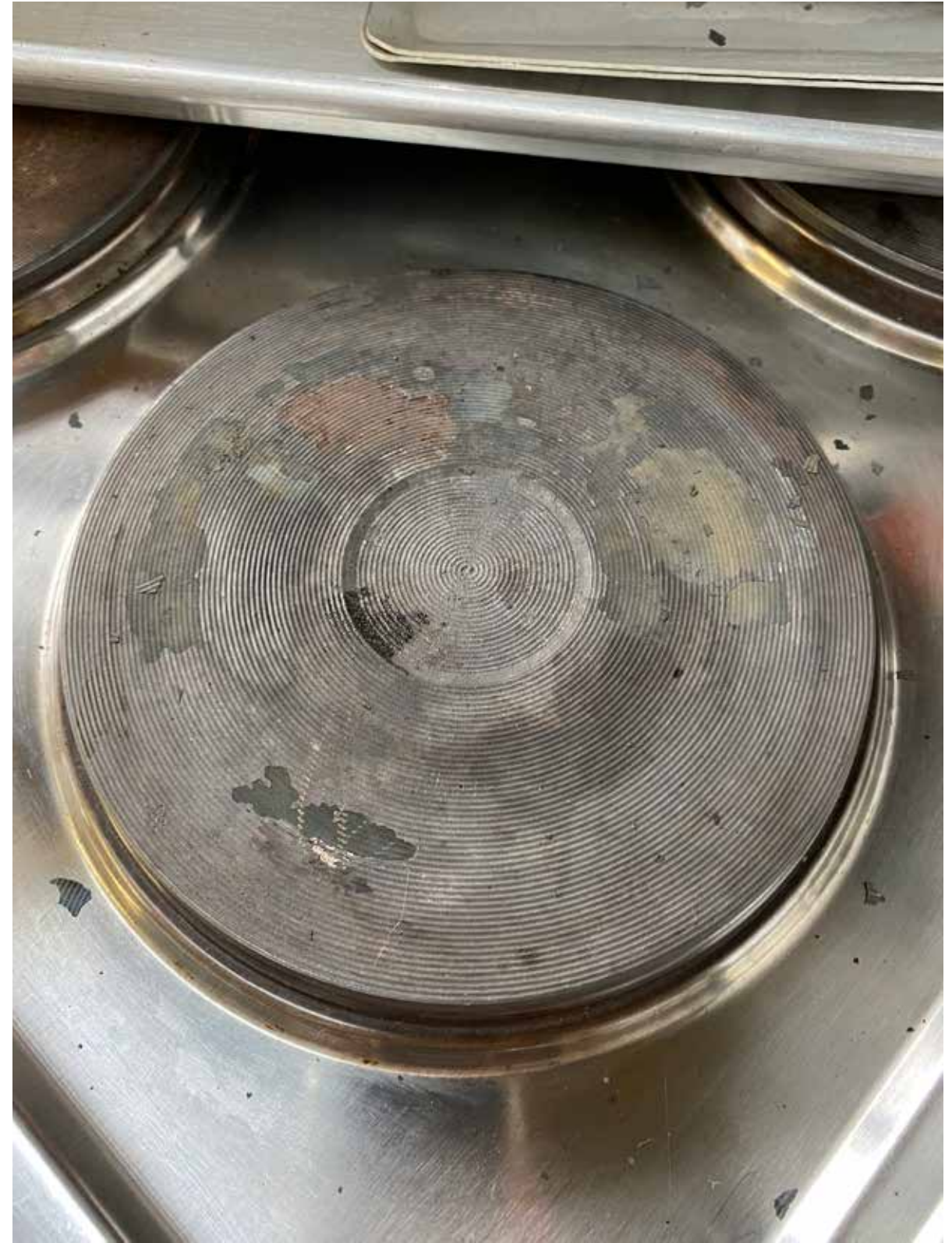
Image 11 Existing hob surface is disintegrating and needs replacing.
