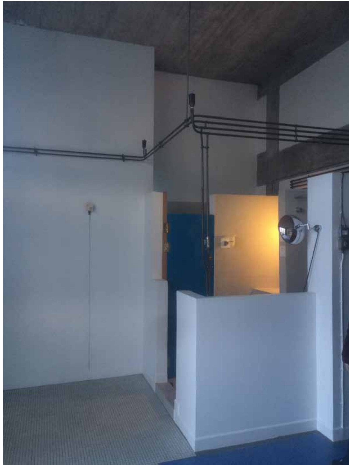
Image 1 Photo showing services crossing wall that prevent any new cupboard being taller than the services.
