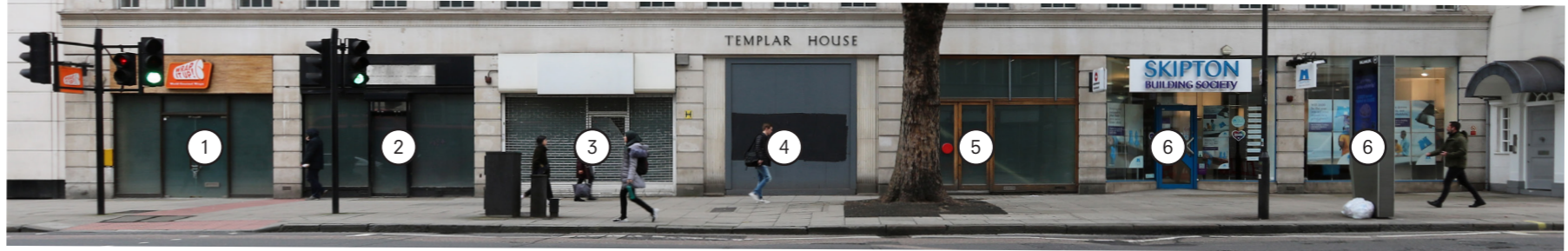
Existing High Holborn Frontage
