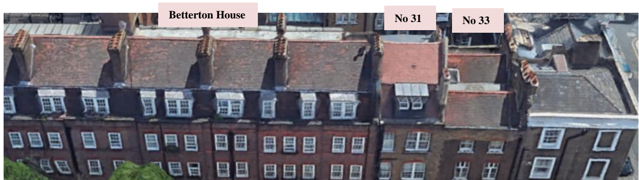
No 33, Roof view front elevation, including Betterton House
