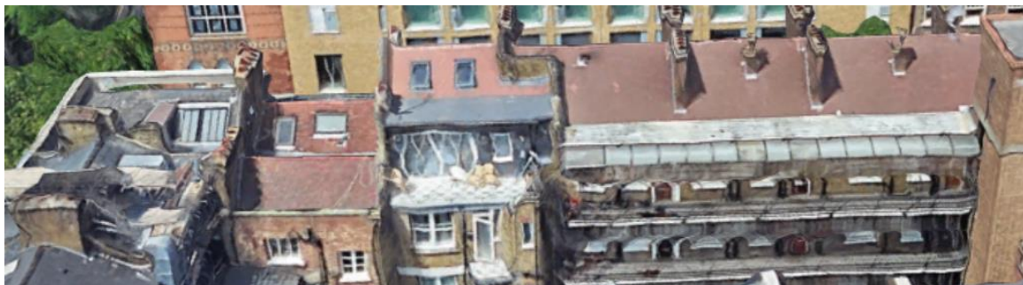
No 33 (and 31, Brownlow House), Roof view rear elevation
