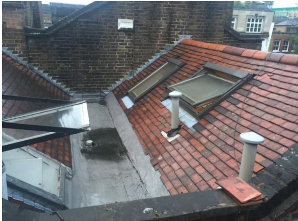
Flat gully between front and rear roof
