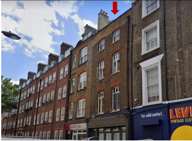
No 33, view from the east at junction with Endell Street
