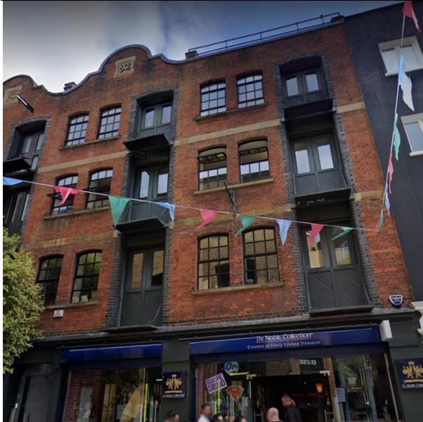
24 Neal Street, hoist doors and iron hoists
