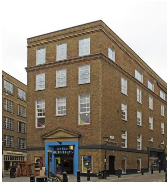
Seven Dials Warehouse, junction of Neal Street, Earlham Street and Shelton Street
