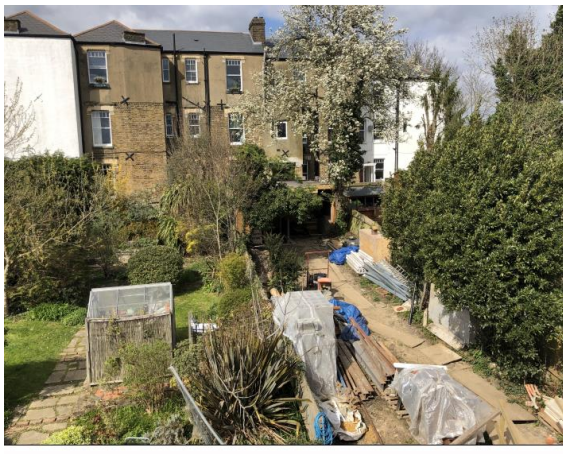
Photo 2: high level view of the rear of the site
