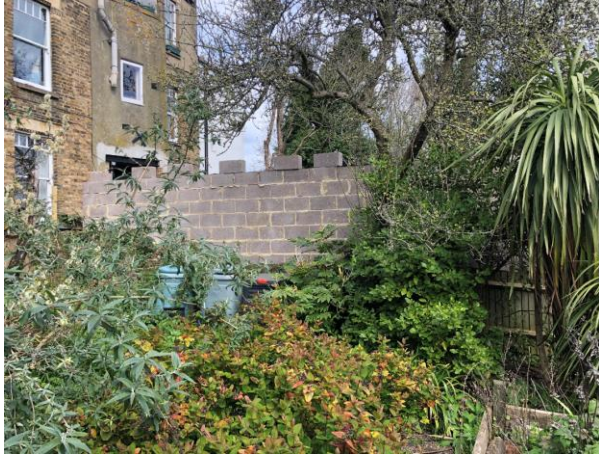
Photo 1: view of shared boundary with no 3, garden typical planting within site
