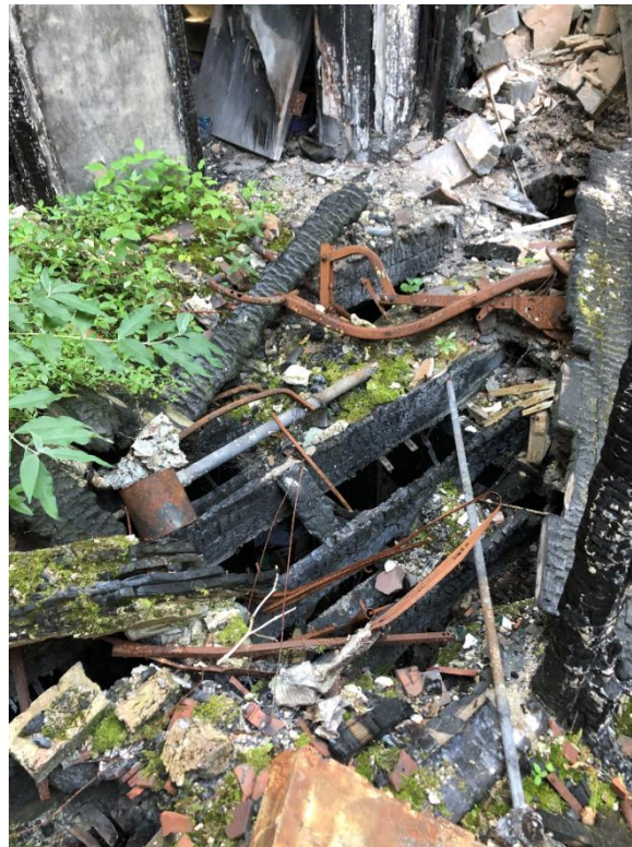
Photo 18 - First floor landing
