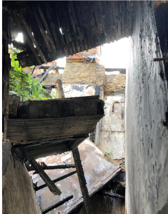
Photo 19 - Apartment 12 view of second floor and roof
