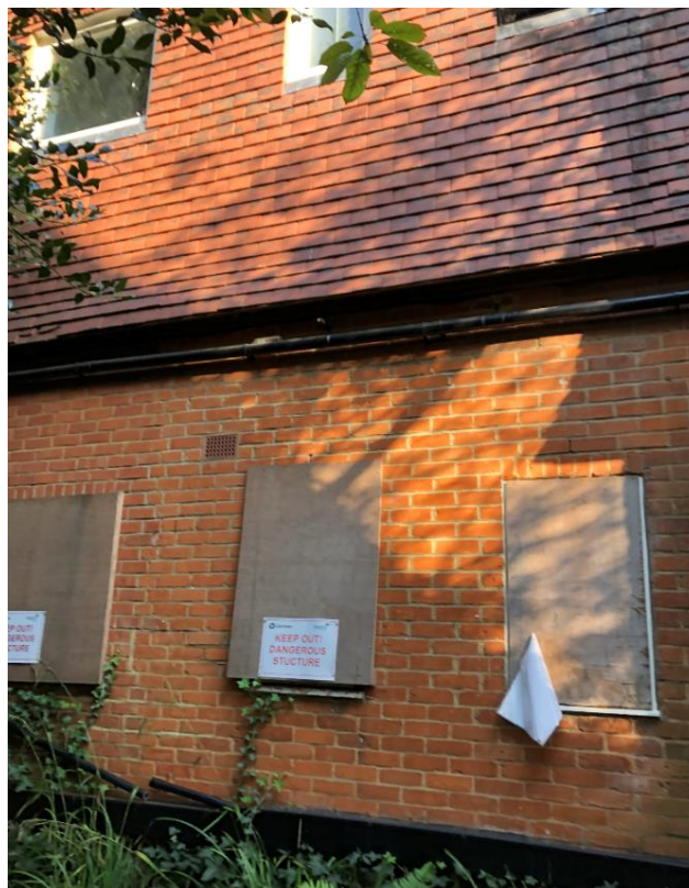
Photo 24 - South side elevation of rear extension
