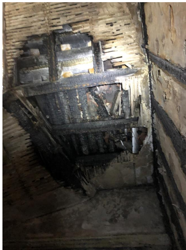
Photo 6 - Apartment 1 bedroom 3 cupboard underside of stair
