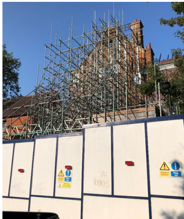
Photo 20 - Front façade gable and scaffold
