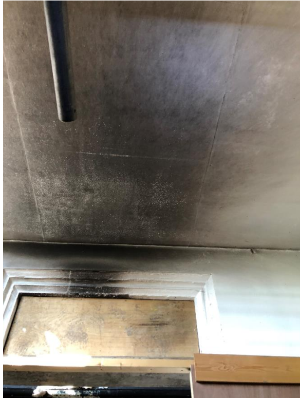
Photo 7 - Main entrance porch
