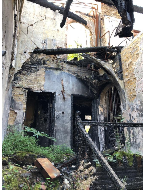
Photo 17 - Stair from ground to first floor
