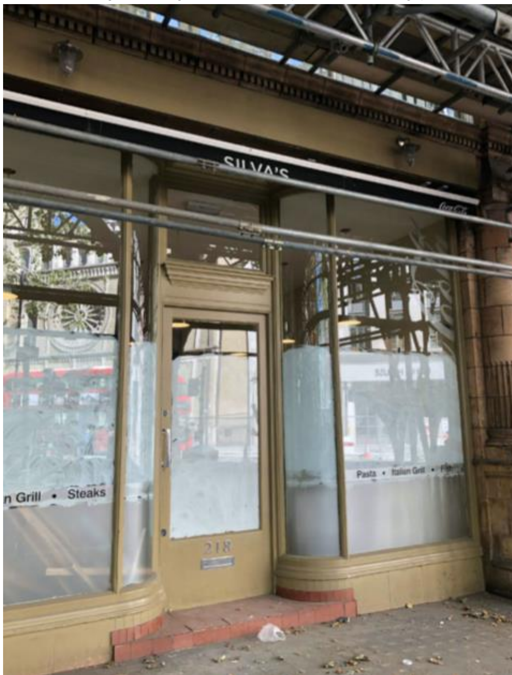
Fig 6 Existing facia of No218 (Source: ZD Design)
