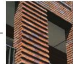
Projecting brick bands
