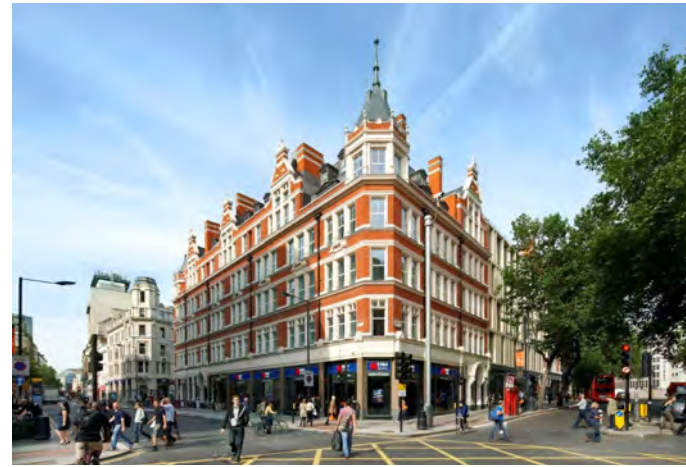
Busy traffic on Southampton Row will hardly be noticeable from the site which is shielded by the frontage properties.
