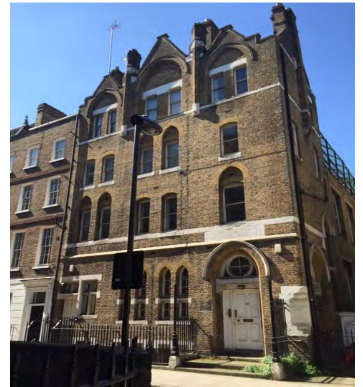
25 Old Gloucester Street from the corner of Queen Square
