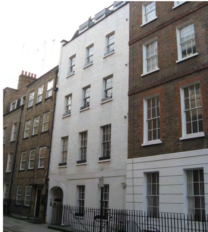
The neighbouring buildings on Old Gloucester Street west side
