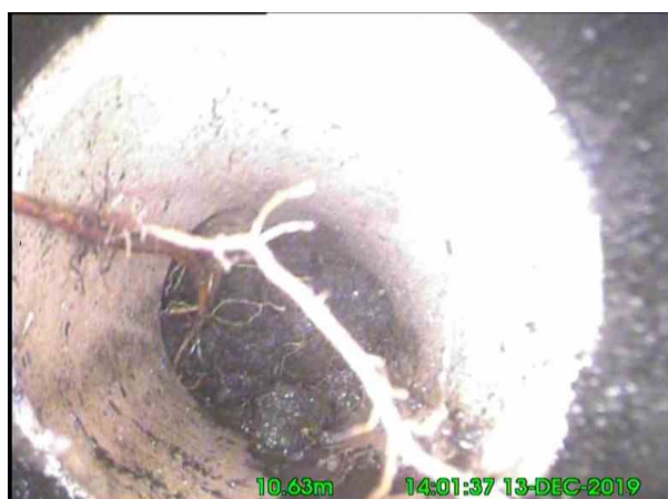
4, 00:01:21, 10.63 m Pipe material changes to vitrified clay at this point
