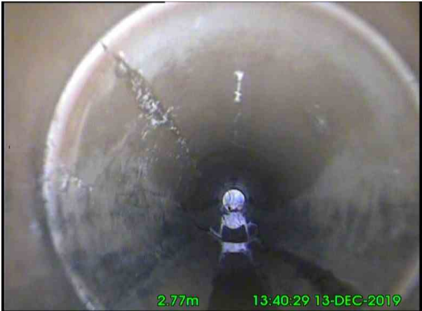
5, 00:00:23, 2.77 m Fracture, longitudinal at joint at 11 o'clock, start
