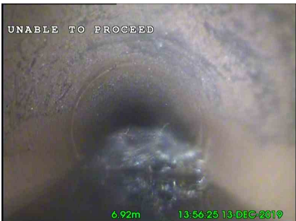
3, 00:01:00, 6.92 m Survey abandoned, UNABLE TO PASS DEBRIS
