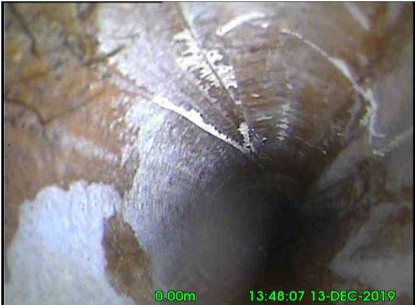
1, 00:00:00, 0.01 m Pipe material changes to epoxy at this point, LINER STARTS
