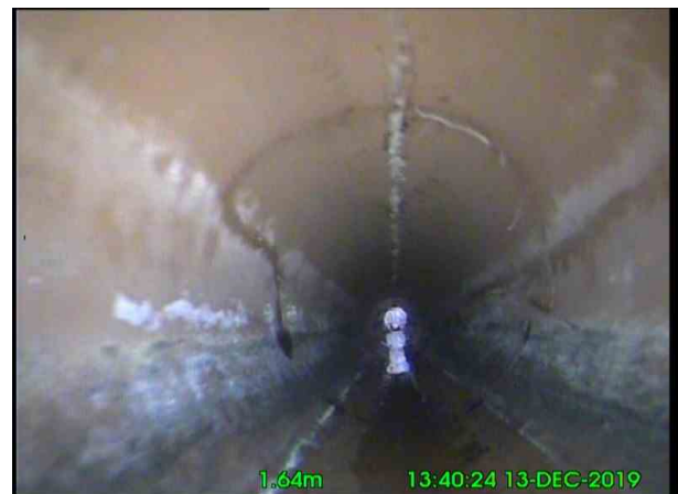
4, 00:00:18, 1.64 m Fracture, circumferential from 9 o'clock to 3 o'clock
