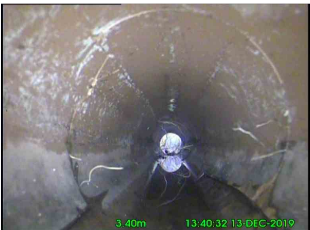
7, 00:00:25, 3.40 m Roots, fine at joint
