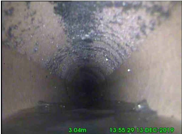
1, 00:00:27, 3.04 m Settled deposits, fine, 5% cross-sectional area loss, start
