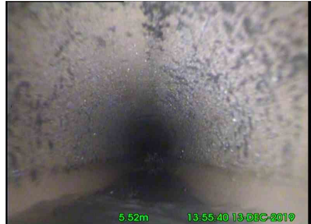
2, 00:00:37, 5.52 m Settled deposits, fine, 5% cross-sectional area loss, start
