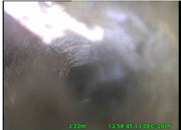
2, 00:00:26, 3.22 m Pipe material changes to epoxy at this point, LINER STARTS
