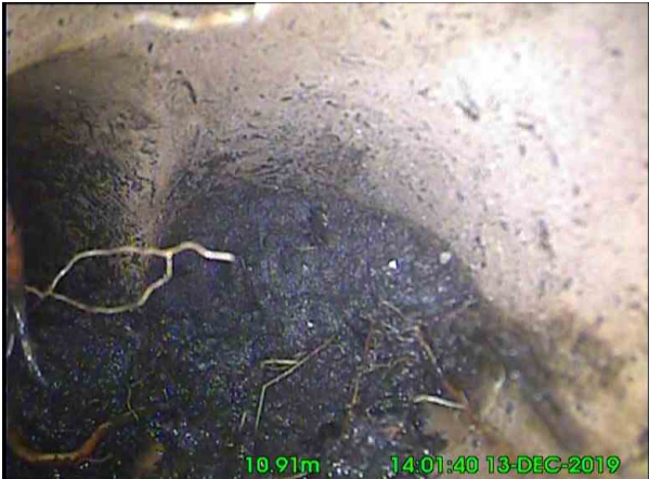
5, 00:01:23, 10.91 m Junction at 9 o'clock, diameter: 100mm
