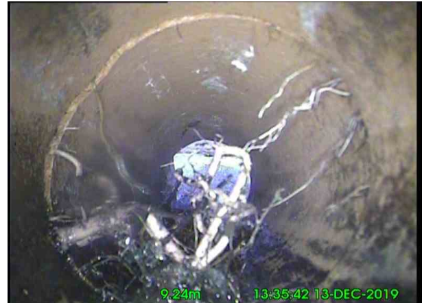
6, 00:00:52, 9.24 m Roots, fine at joint
