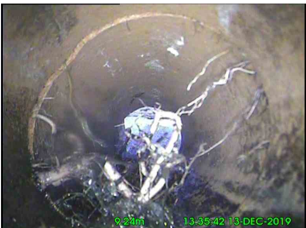
7, 00:00:52, 9.24 m Deformed sewer or drain, 10%
