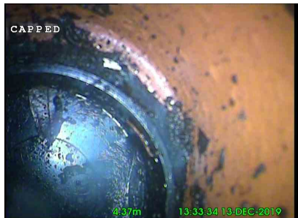
4, 00:00:45, 4.37 m Finish node type, major connection without manhole, reference number: CAPPED OFF
