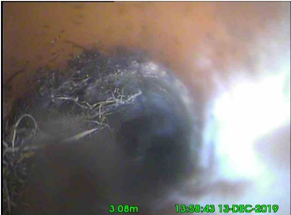
1, 00:00:24, 3.08 m Roots, mass at joint, 10% cross-sectional area loss
