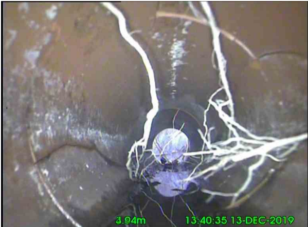
9, 00:00:29, 3.94 m Fractures, multiple from 12 o'clock to 12 o'clock
