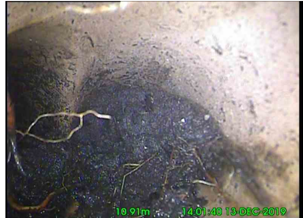
6, 00:01:23, 10.92 m Settled deposits, fine, 100% cross-sectional area loss, SILT
