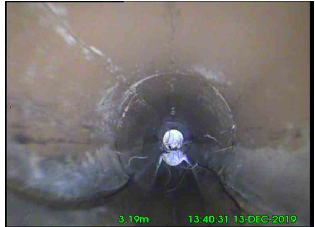
6, 00:00:24, 3.19 m Fracture, longitudinal at 5 o'clock, start
