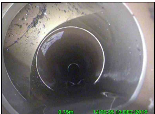
1, 00:00:18, 0.75 m Junction at 10 o'clock, diameter: 100mm
