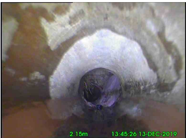
3, 00:00:22, 2.15 m Fracture, circumferential from 7 o'clock to 3 o'clock
