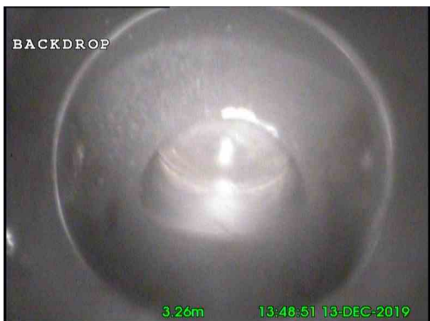
3, 00:00:42, 3.24 m Finish node type, manhole, reference number: CWMH 05, IN BACK DROP
