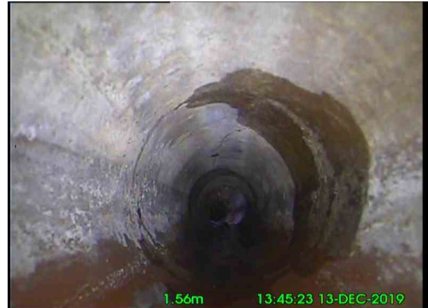
2, 00:00:18, 1.56 m Fracture, longitudinal at joint at 12 o'clock, start
