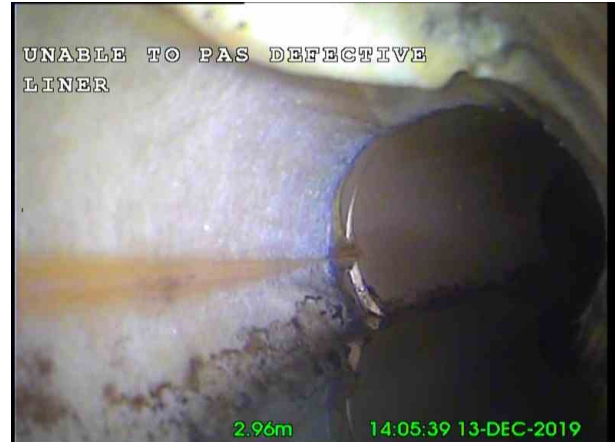
6, 00:01:10, 2.96 m Survey abandoned, UNABLE TO PASS DAMAGE LINER
