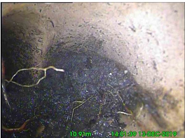
7, 00:00:00, 10.95 m Survey abandoned, UNABLE TO PASS DEBRIS
