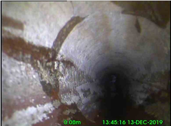
1, 00:00:12, 0.01 m Fracture, circumferential from 7 o'clock to 12 o'clock
