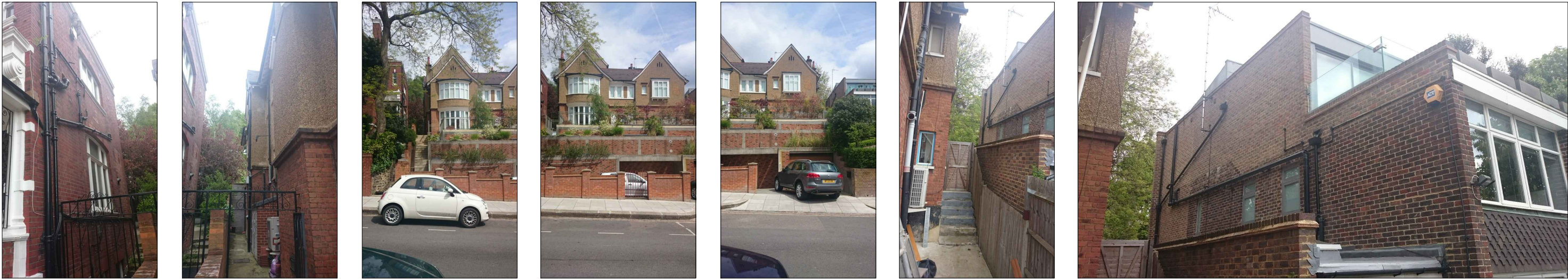
FRONT ELEVATION PHOTOS
