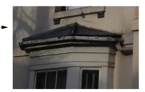
Cement render covering the flashing to be removed a 35mm upstand to the wall abutment used for the wood roll detail, a cover flashing bossed to cloak the meeting point of the two ridge rolls where they meet at the wall. Head fixings must be sealed prior to the cover flashing. Roman cement used to repair render to the cover flashing (lead wedges @450mm ctrs) no render used over flashing (note failure of render and damp ingress in existing detail).
