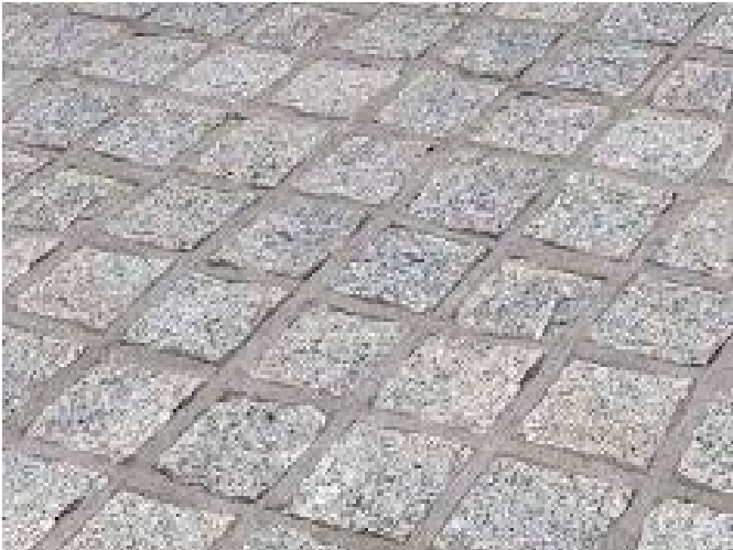
Granite setts to be used as edging detail
