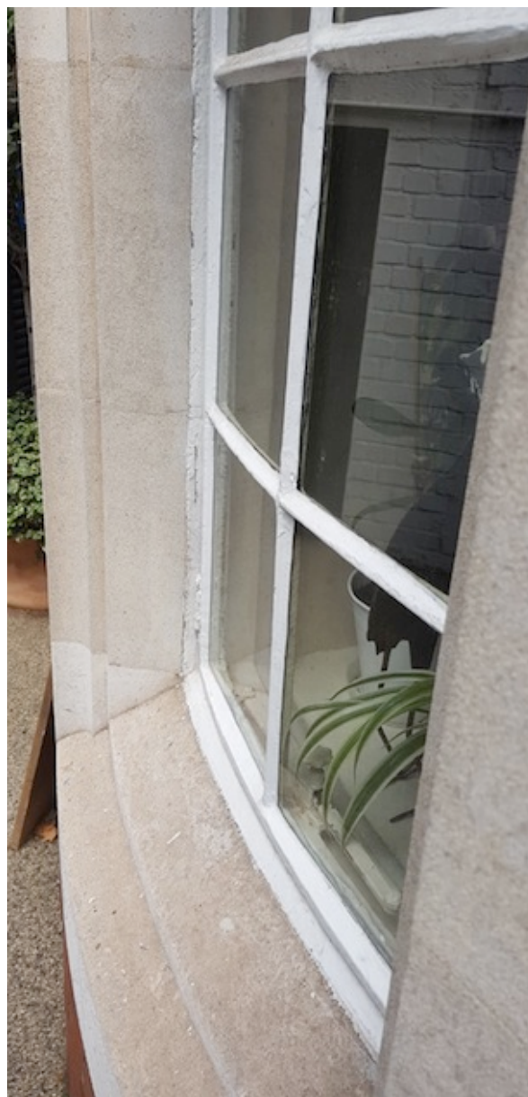
12 Bloomsbury Street – New flat window frames, double-glazed
