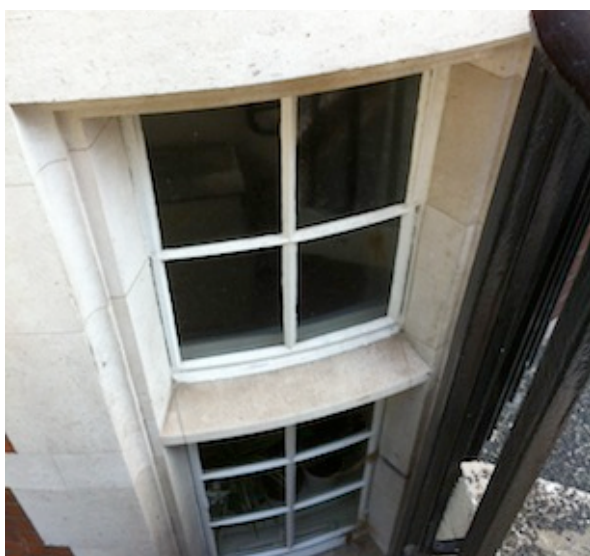
12A Adeline Place – Original curved window frames, single-glazed with curved glass ▲ ►
