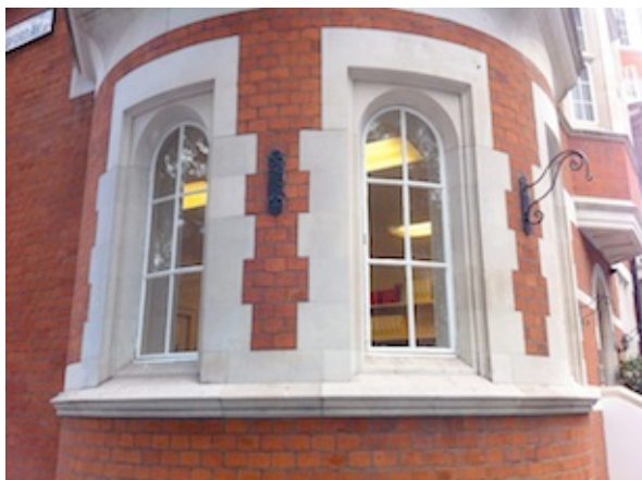
12 Adeline Place – Original curved window frames, single-glazed
