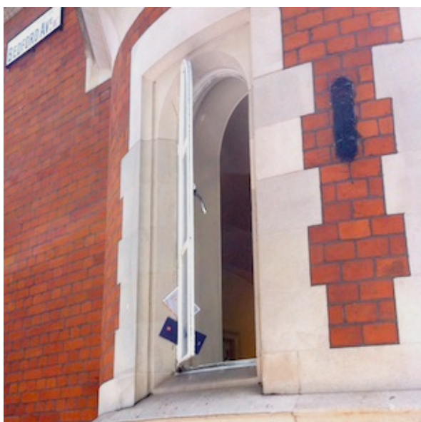
12 Adeline Place – Original curved window frames, single-glazed
