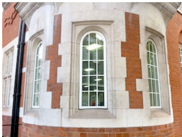
12 Bloomsbury Street – New flat window frames, double-glazed
