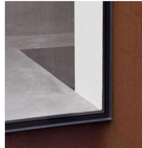
Precedent images of Corten cladding and minimally framed glazing adjacent to traditional brickwork / openings
