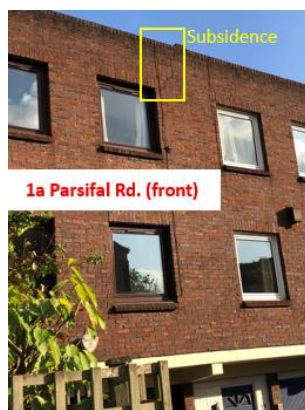
Figure 1.1 - Front of 1a Parsifal Road
