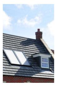
Solar water heating systems use free heat from the sun to warm domestic hot water. Solar hot water heating can generate a large proportion of a dwelling's annual DHW requirement. The displaced fuel would be mains gas meaning that the CO<sub>2</sub> savings of this type of system would be relatively low due to the low carbon intensity of the displaced fuel.
