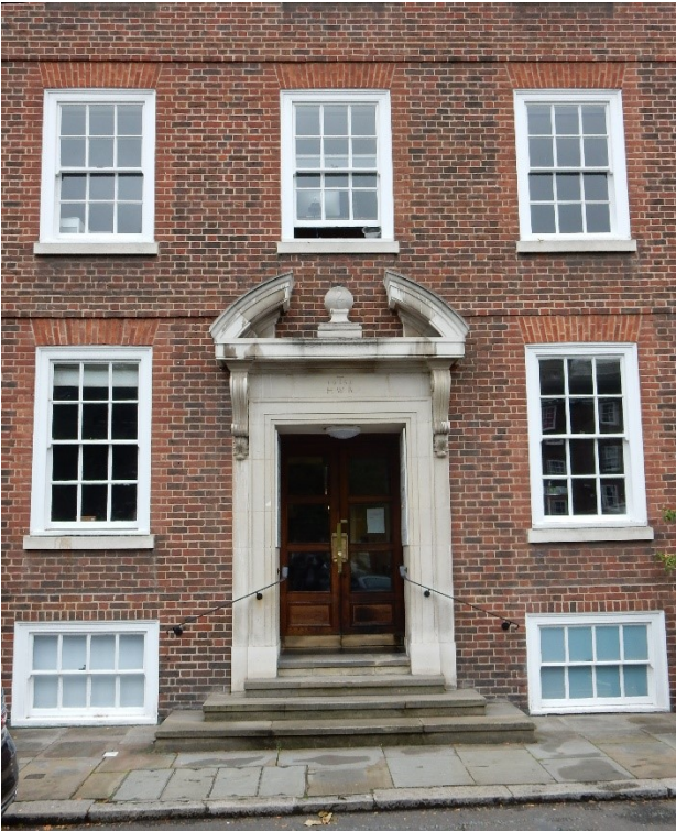
No 2 Entrance showing external steps to front door
