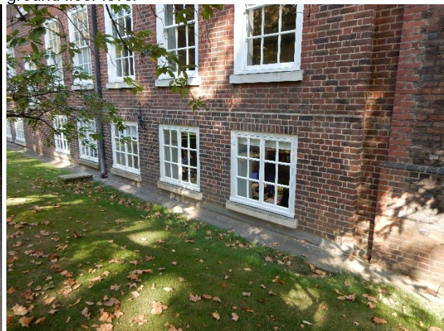
No 2 Rear Elevation showing asphalted drainage channel below basement windows
