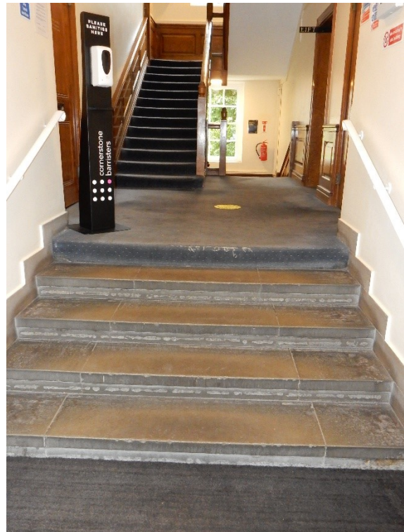
No 2 Entrance level showing internal steps to raised ground floor level
