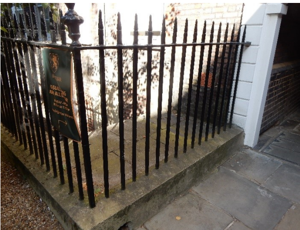
Attached railings to rear of No 1 Gray's Inn Square
