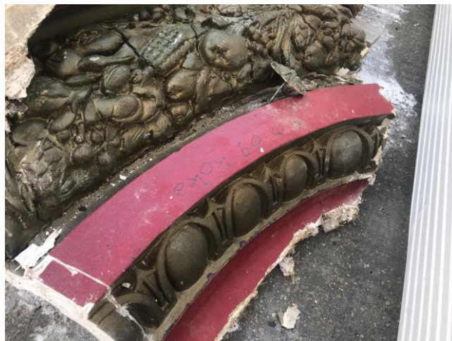
e. Circular beam case with egg and dart moulding, B.
