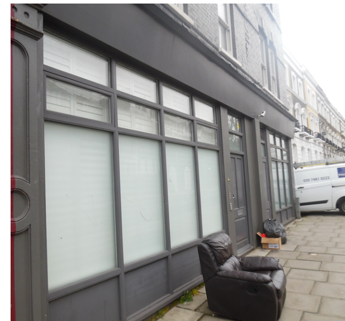
Photo of no. 19 Fortess Road
