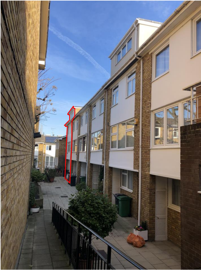
3. View towards 38 Meadowbank from upper level
