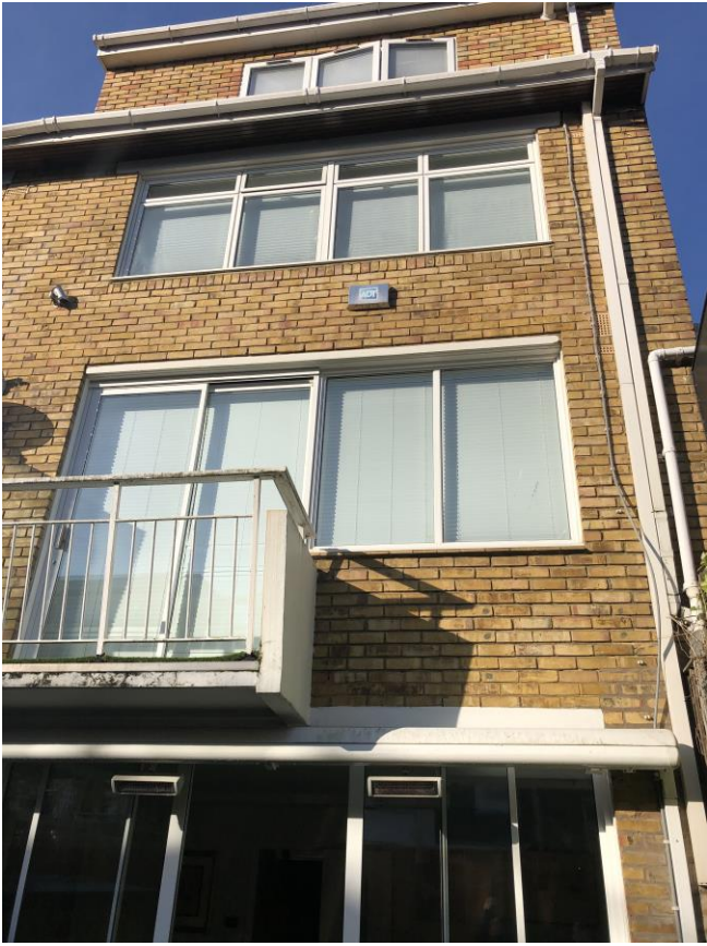
7. View of rear elevation of 38 Meadowbank
