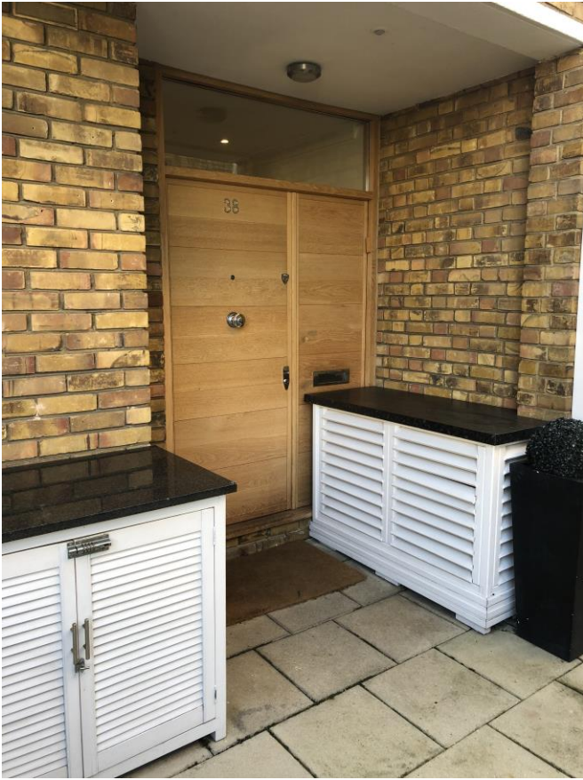
5. Entrance of 38 Meadowbank with existing louvered enclosure for air conditioning condenser
