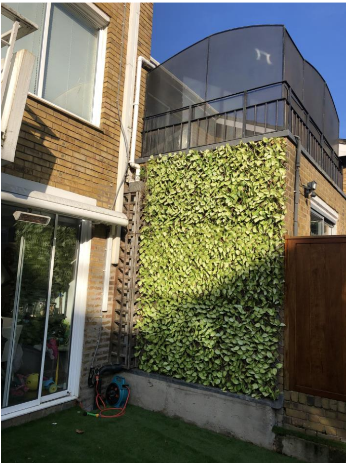
6. View of rear of 38 Meadowbank and flank wall and upper floor terrace of no. 39
