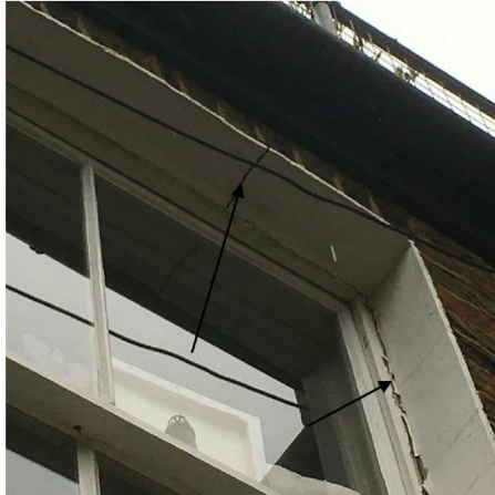
Cracking at the mid length of the flank wall of the back addition
