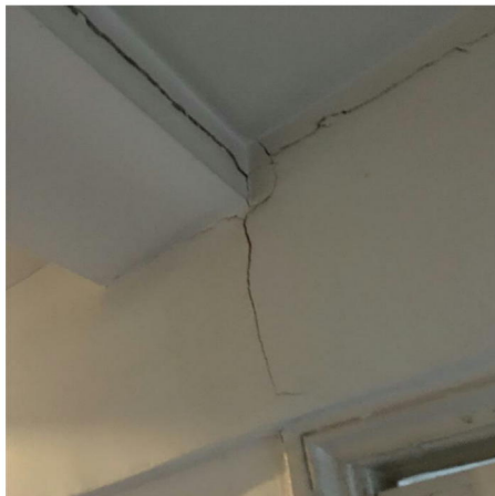
Cracking on the first floor landing
