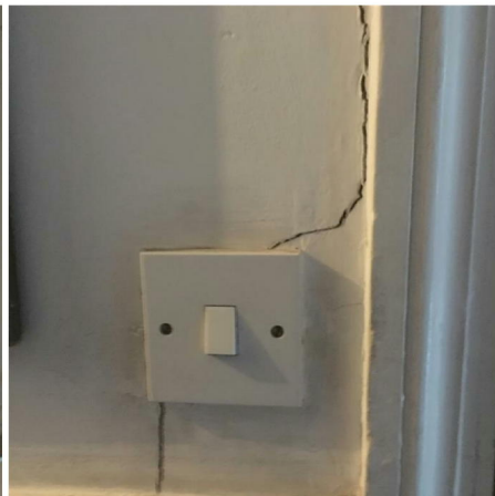
Cracking on the first floor landing
