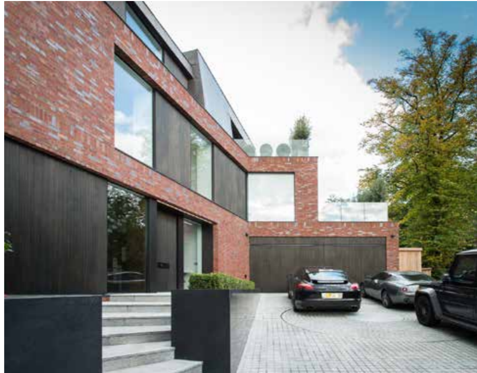
1 - Front driveway currently used for parking instead of garage
