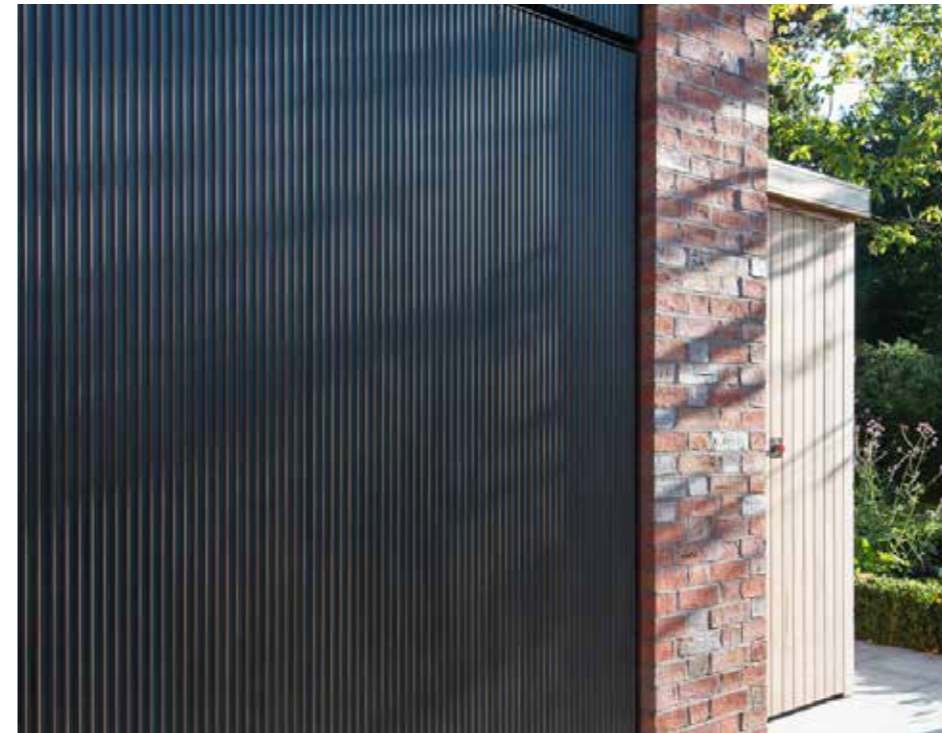
4 - Existing garage door and side storage
