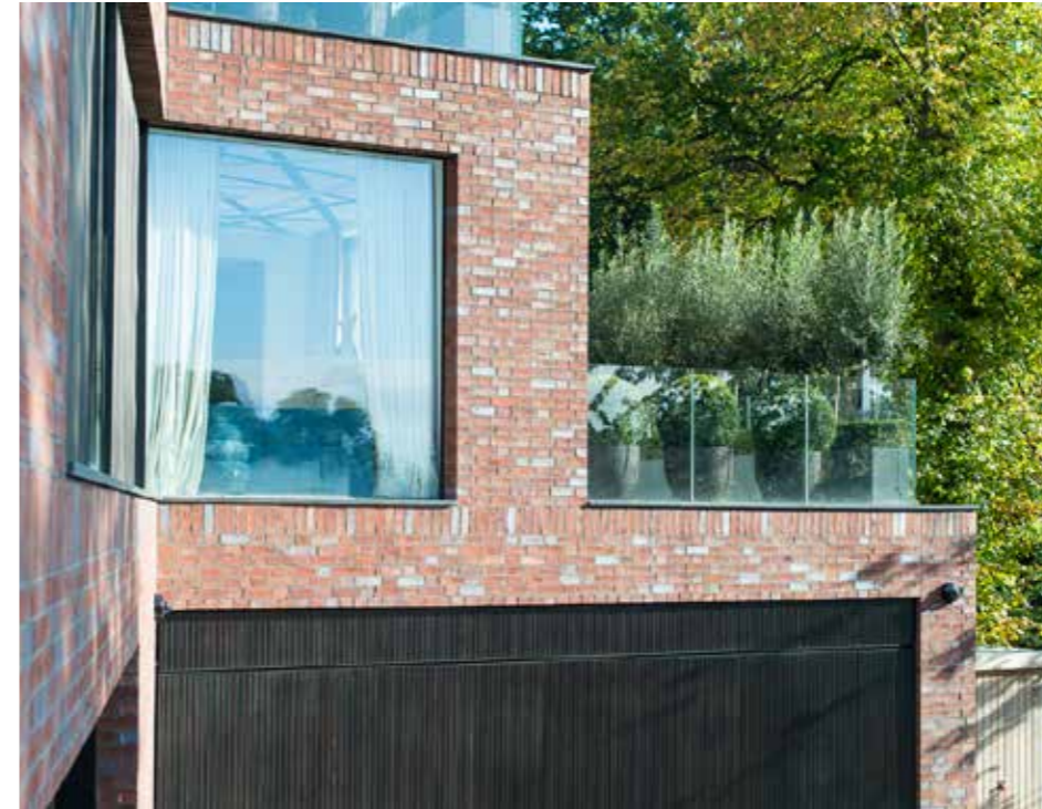
2 - Existing garage door with front facing balcony
