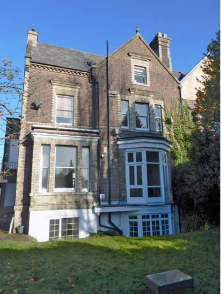
e) view of existing rear elevation of house *
