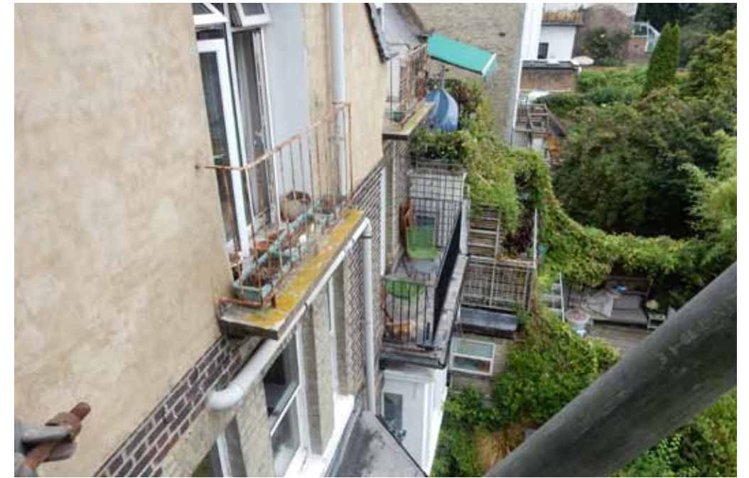
k) multiple balconies at rear of adjoining property at no 31
