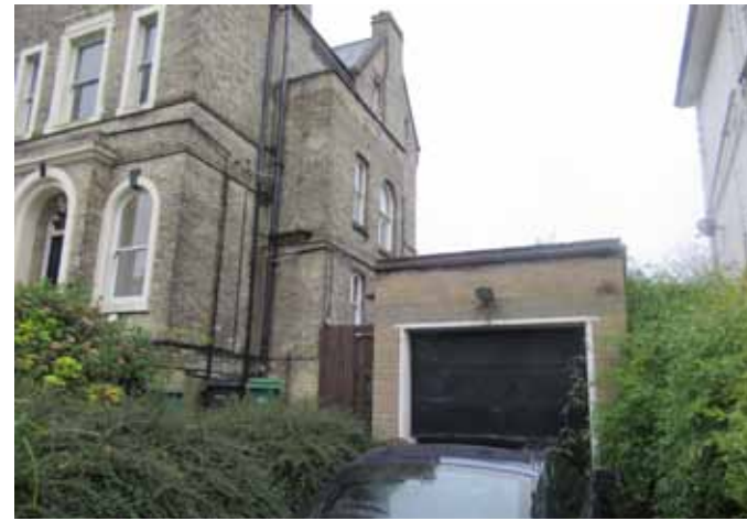
j) gap to no 35 from eye-level on street with garage obscuring views to rear
