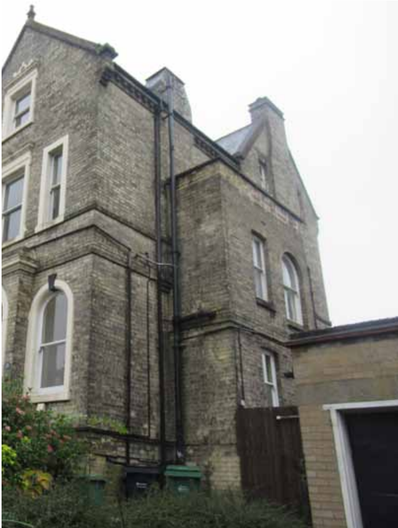
d) view of existing flank elevation of house *
