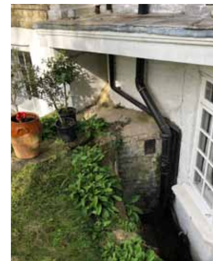
r) vented void infill to rear areaway to be removed, with existing projecting platform above
