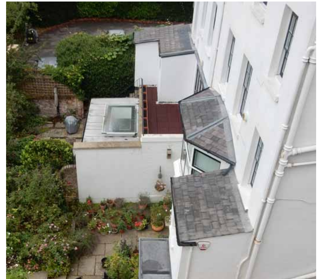
l) view of extensions nos 35 & 37 showing upper ground floor level full width balcony at no 37
