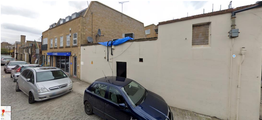
317-319 Kentish Town Road (existing single storey to York Mews benefiting from planning permission) 6-8 York Mews (blue sign) 10 York Mews (Juliette balcony)
