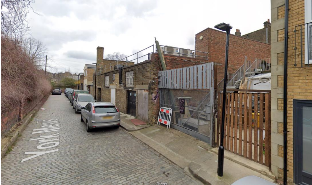
327 Kentish Town Road (no built form to York Mews) 329-331 Kentish Town Road (application site)
