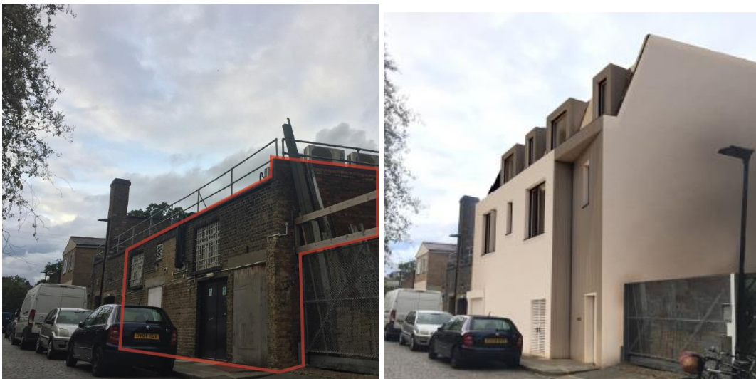
Images – showing the existing and proposed treatment of the York Mews frontage
