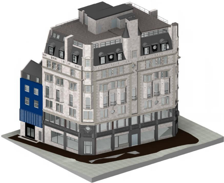
Erection of the façade retention scheme
