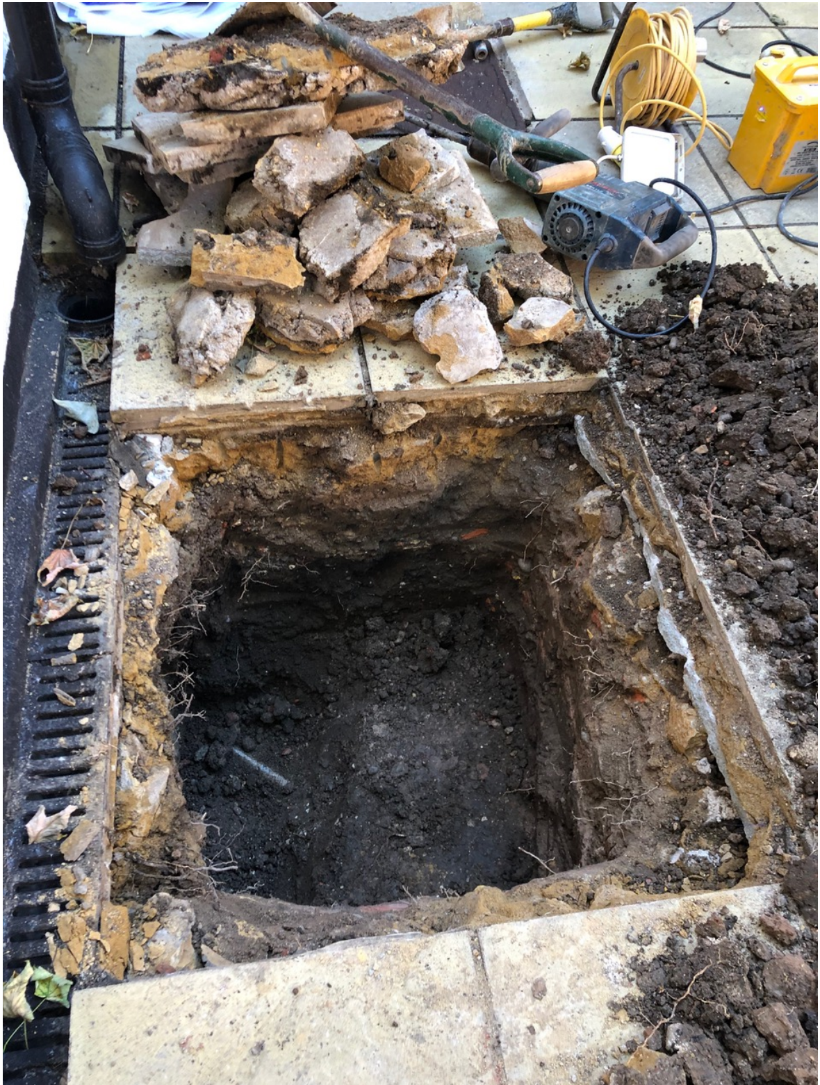
Photograph A2.1: No significant rooting in trial pit
