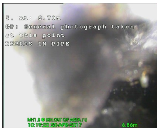
, 00:00:37, 6.88m General photograph taken at this point DEBRIS IN PIPE
