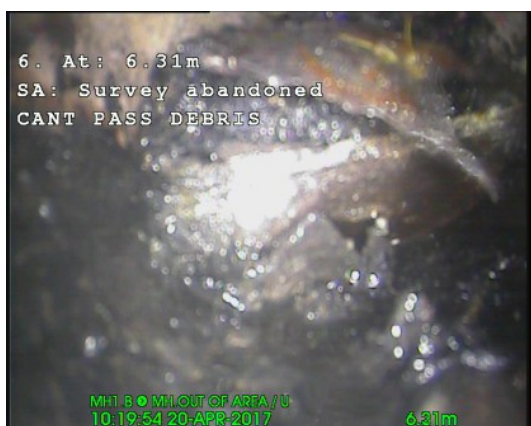
, 00:00:52, 6.19m Survey abandoned CANT PASS DEBRIS
