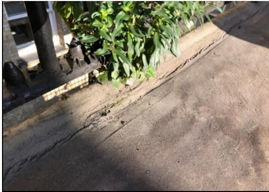
Photograph No. 9 Trees have taken root in the upstands.
