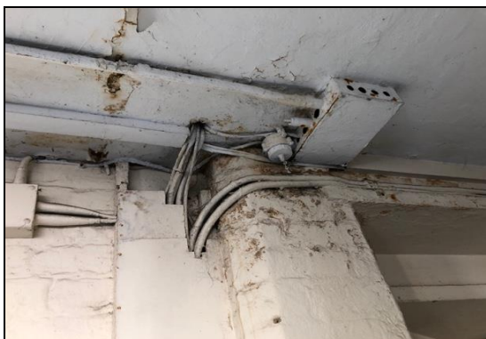
Photograph No. 12 Ingress can be seen on the lower floors indicating the walkways require attention.
