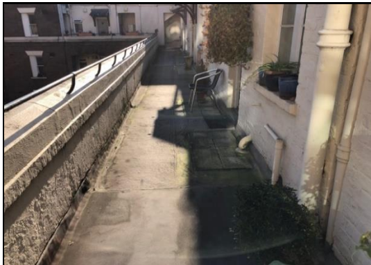
Photograph No. 10 Walkways – the original asphalt covering has been overlaid with a liquid covering indicating a history of ingress.
