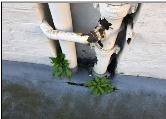
Photograph No. 11 Plants have taken root in the splits and penetrations of the asphalt.
