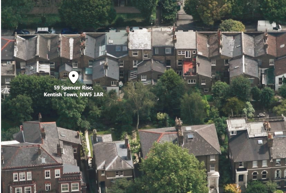
Photo 7 – Rear elevation of Spencer Rise properties (Chetwynd Road properties bottom of image)
