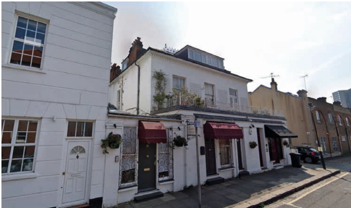
Fig 11: Lambolle Place looking east at no. 18 and Lancaster Garages
