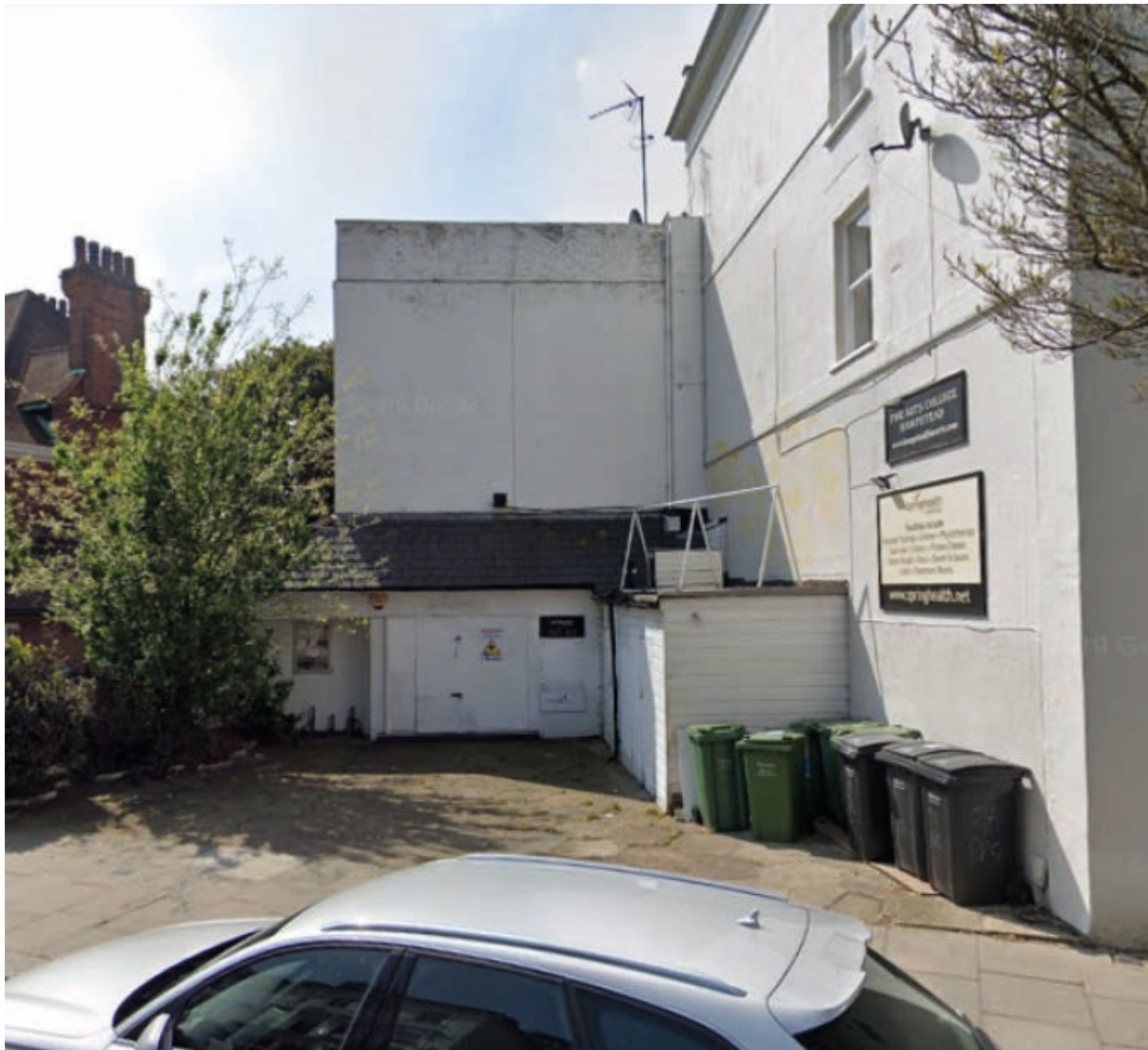
Fig 1: Entrance elevation - view from Belsize Park Gardens looking south west
