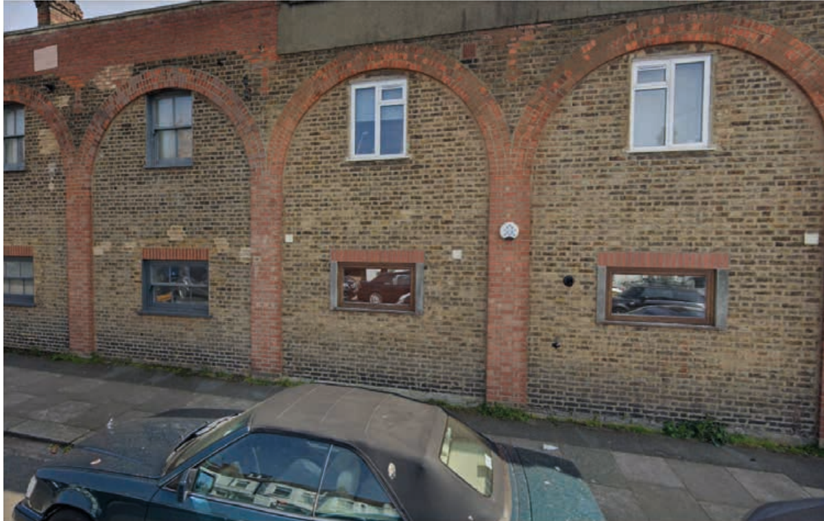
Fig 10: Lambolle Place looking east to Eton Garages
