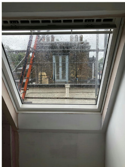
View from landing showing AOV without Privacy Film and after it has been fitted
