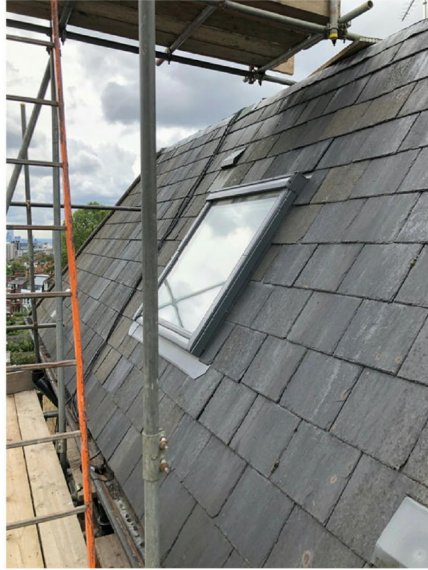
Close Up - Installed AOV and projection (80mm) from roof
