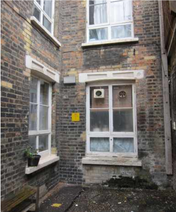
Window type W3, side-hung casements over fixed lights
