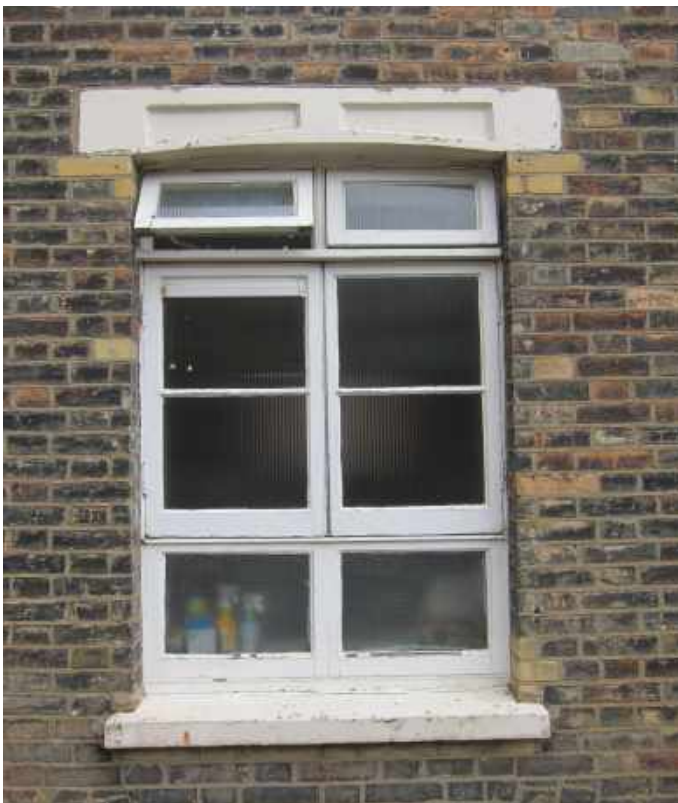
Window type W2, side-hung casements below top-hung ventilator lights
