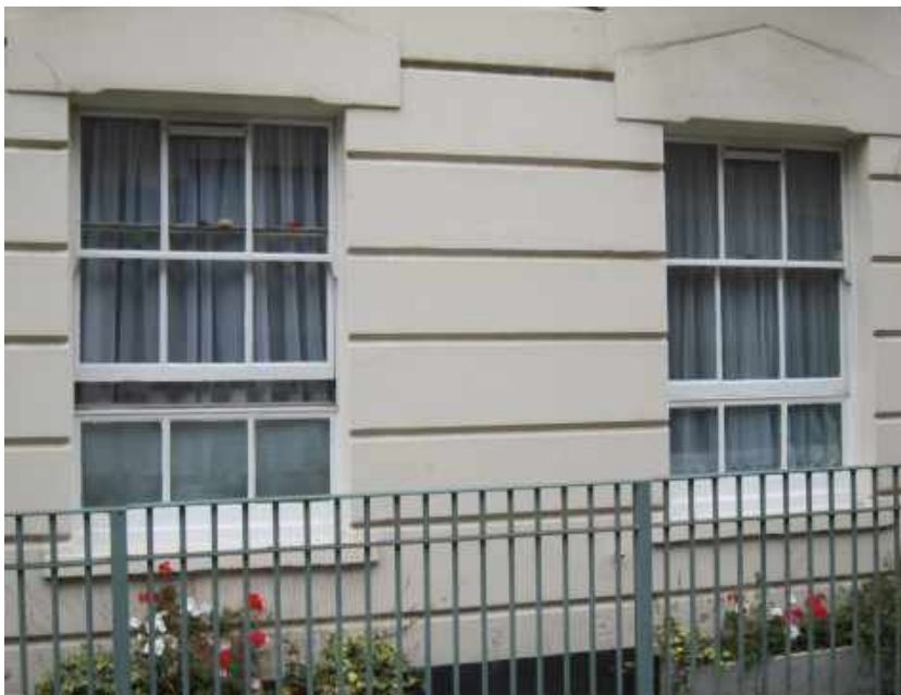
Typical front elevation sash windows: repairs only proposed
