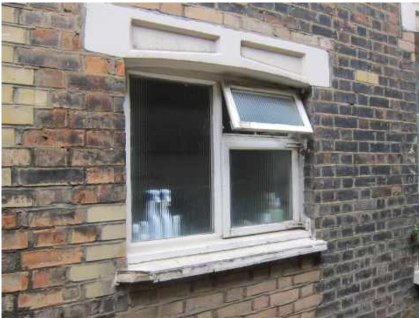
Window type W7, side-hung casement below top-hung ventilator light
