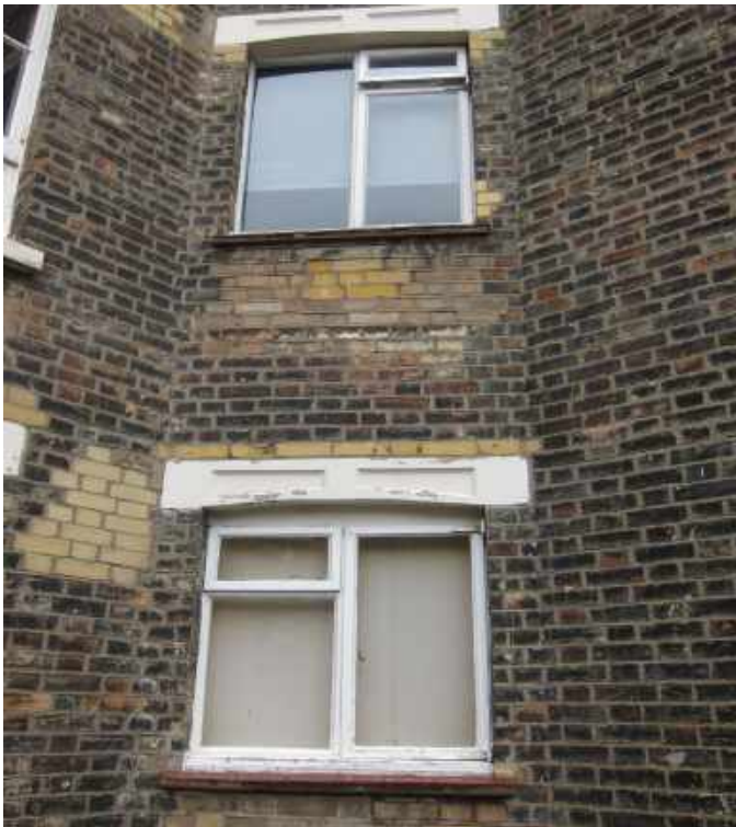
Window type W5, side-hung casement with small top-hung ventilator over and fixed light adjacent, above type W8, side-hung casement with small top-hung ventilator over fixed light
