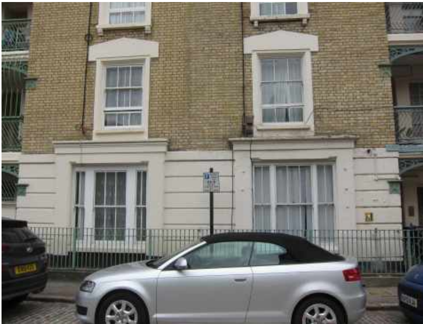
Part front elevation showing mullioned sash windows
