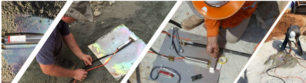
Figure 2 - Settlement Plates being installed
