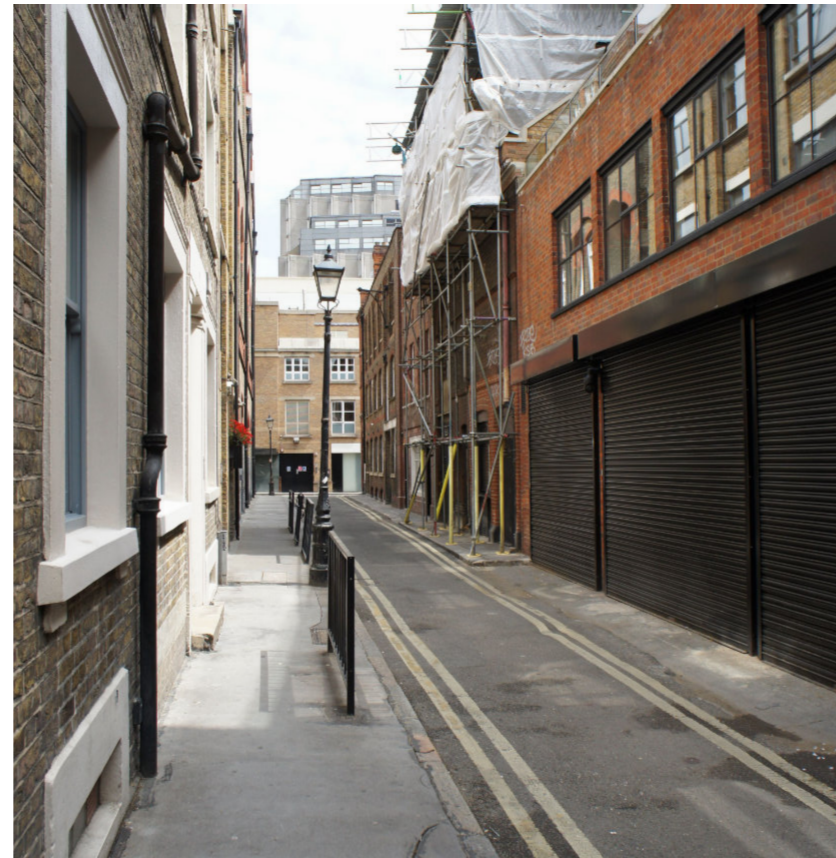
Photograph - Hanway Place looking east
