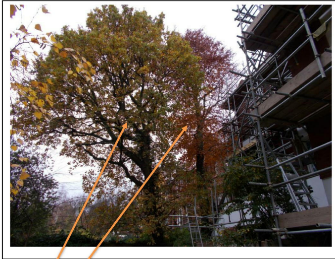
View of T2 and T1
