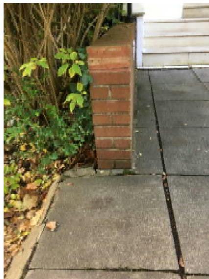
Rotation of dwarf wall at entrance
