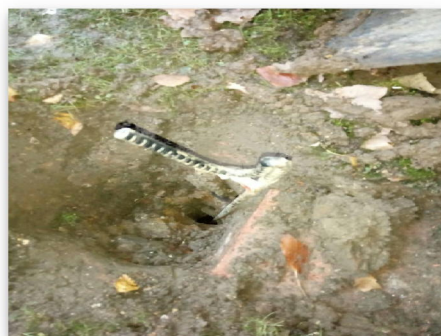
Fig 1.2: Trial Hole 1 Footing
