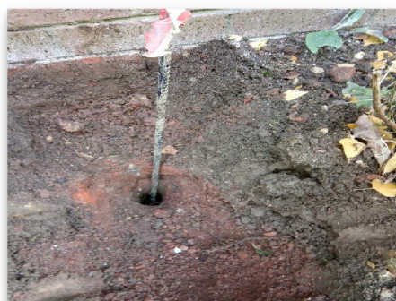
Fig 2.2: Trial Hole 2 Footing
