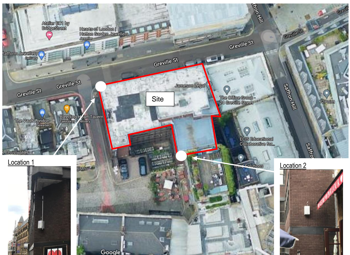
Figure 1 Construction Monitoring Locations
