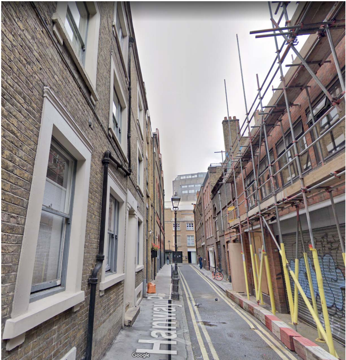
Figure 2: site photograph showing unusually narrow width of Hanway Place, restricting sky visibility
